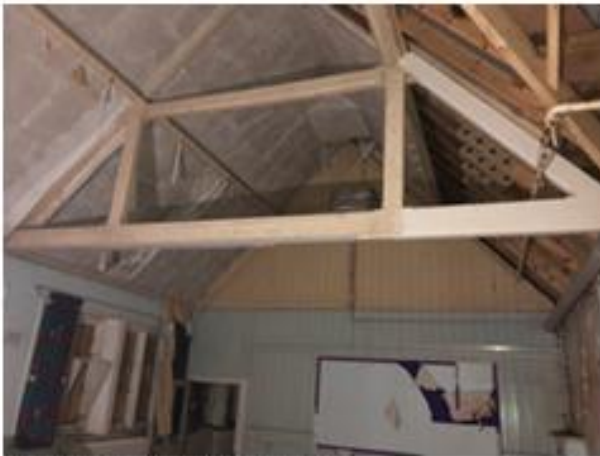
School Interior roof structure
