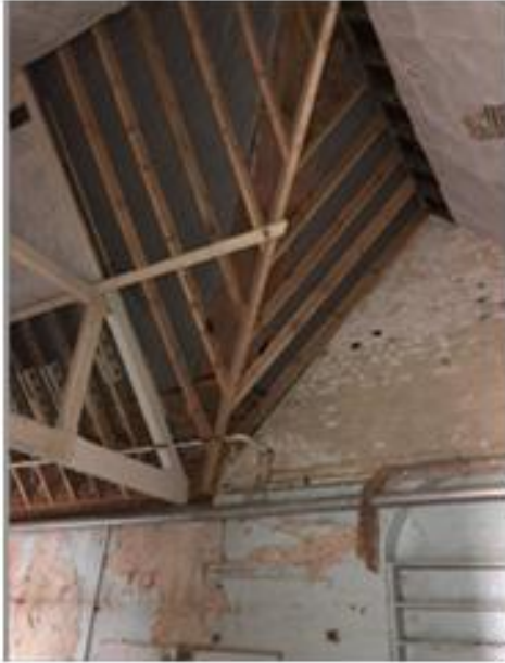
School Interior roof structure
