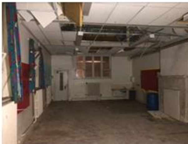
School Interior facing East to external wall
