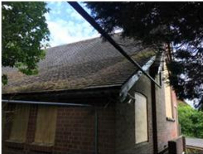
Rear East and South facades.
