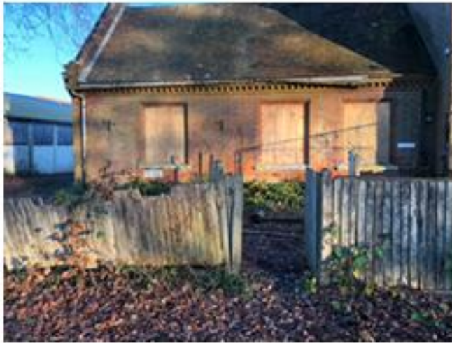
Front west façade
