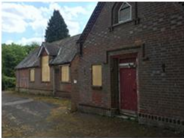
Side North façade
