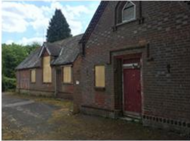
Side North façade
