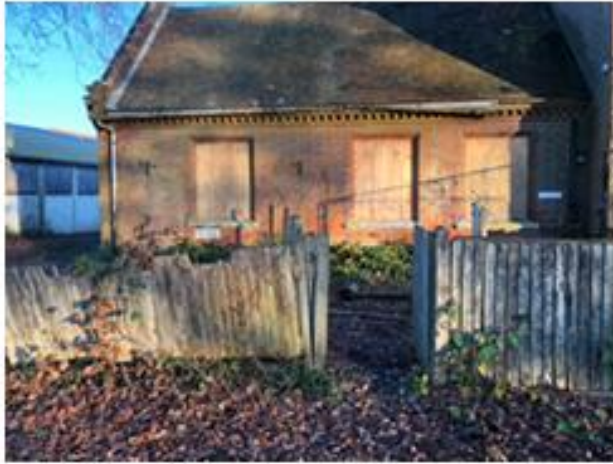
Front west façade
