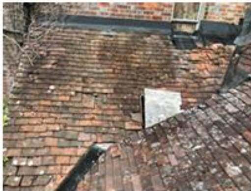
Roof junction with rear of house.
