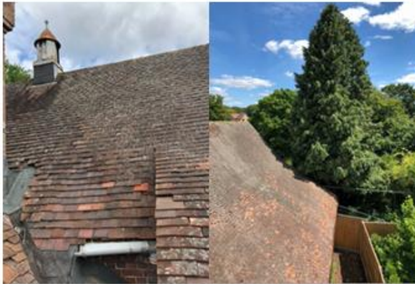
Existing school roof condition: Facing south
